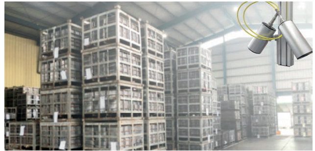
Monitoring of a storage hall
